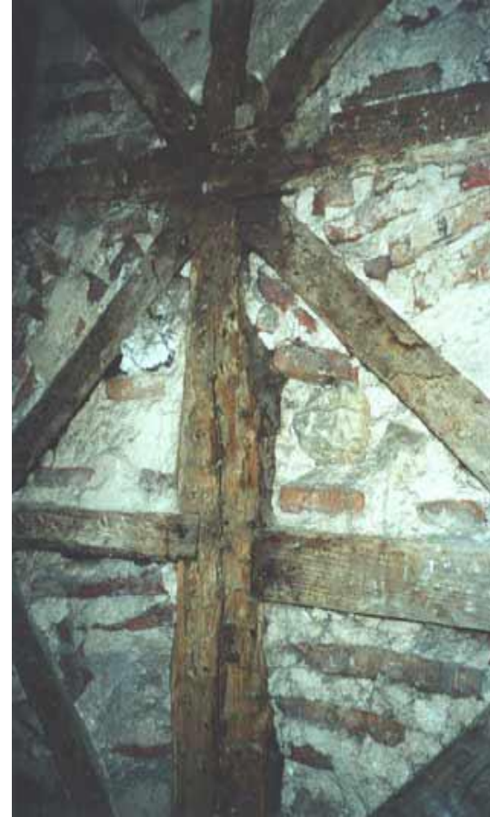
Gaiola Pompalina: Three dimensional wooden structure in masonry walls
