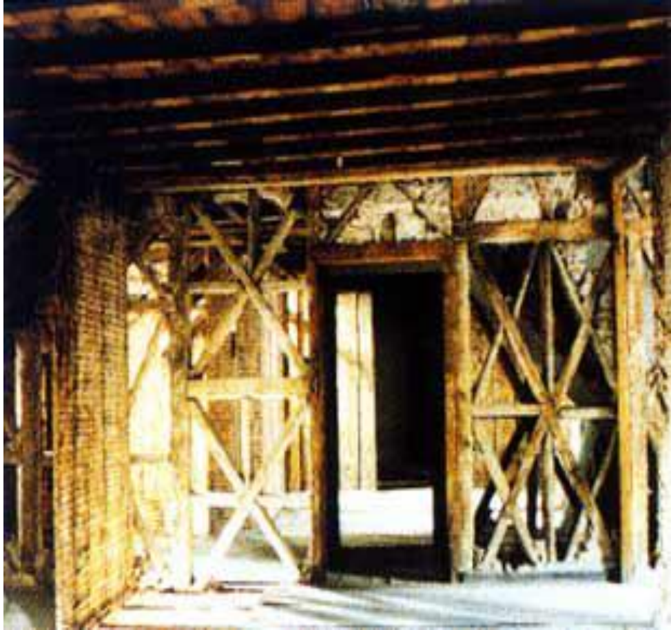
Gaiola Pompalina: Three dimensional wooden structure in masonry walls
