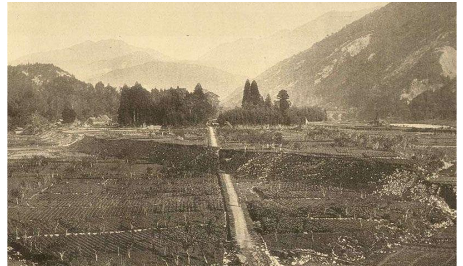
“The Neo Fault”
